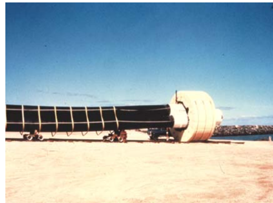
Figure 4. The upper portion of the “OTEC 1” CWP being pulled into Kawaihae Harbor, Hawaii
