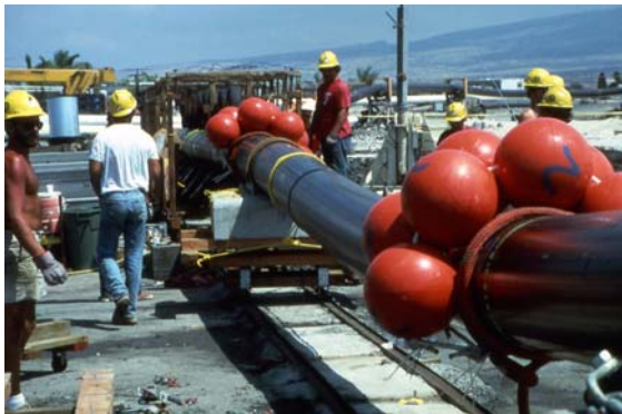
Figure 2. Deployment of a 0.45 m (18”) diameter CWP (photo courtesy of Makai Ocean Engineering, Inc.)
