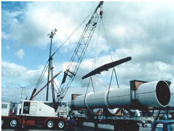
Figure 5. A 24 m section of the 2.5 m diameter FRP CWP tested off of Honolulu in 1983
